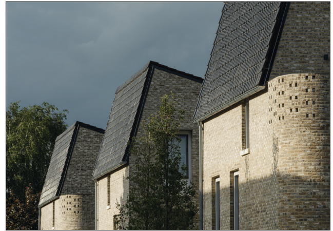
The unique roofing system flows without interruption continuously from eave to ridge.
